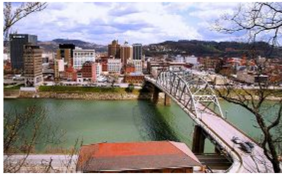
South Side Bridge, Charleston, W. Va. as it looks today.
